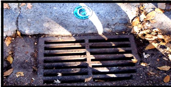
**Storm Drains** are roadside grates that collect rainwater from streets, sidewalks, and parking lots and empty it into rivers, lakes and groundwater.
